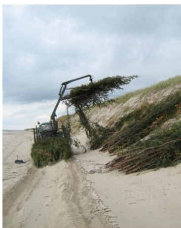
Figure 3.3 Maintenance of foredune ridge after a storm event.
